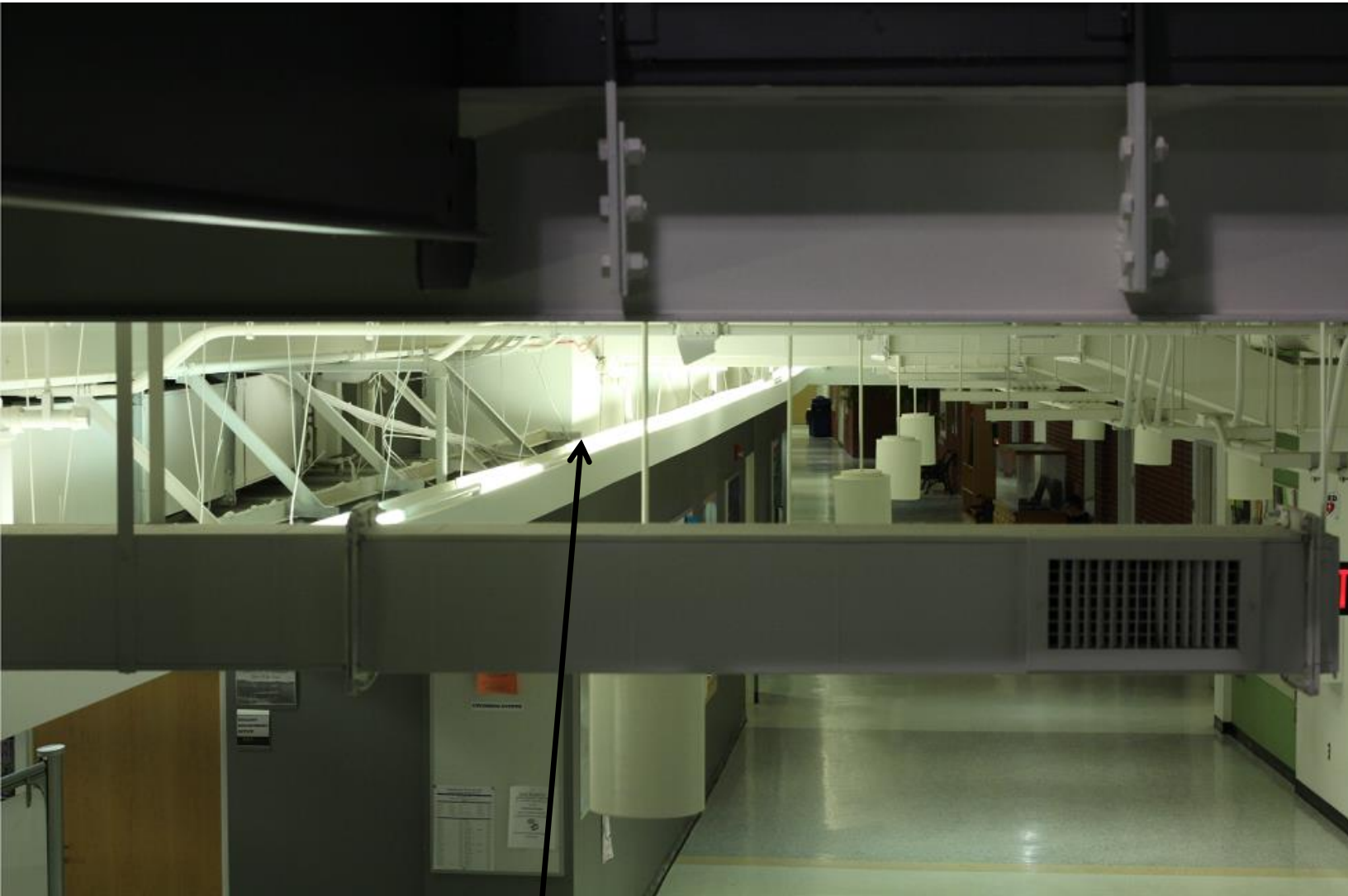
Tube-lights illuminating ceiling tucked above vents in Magruder
